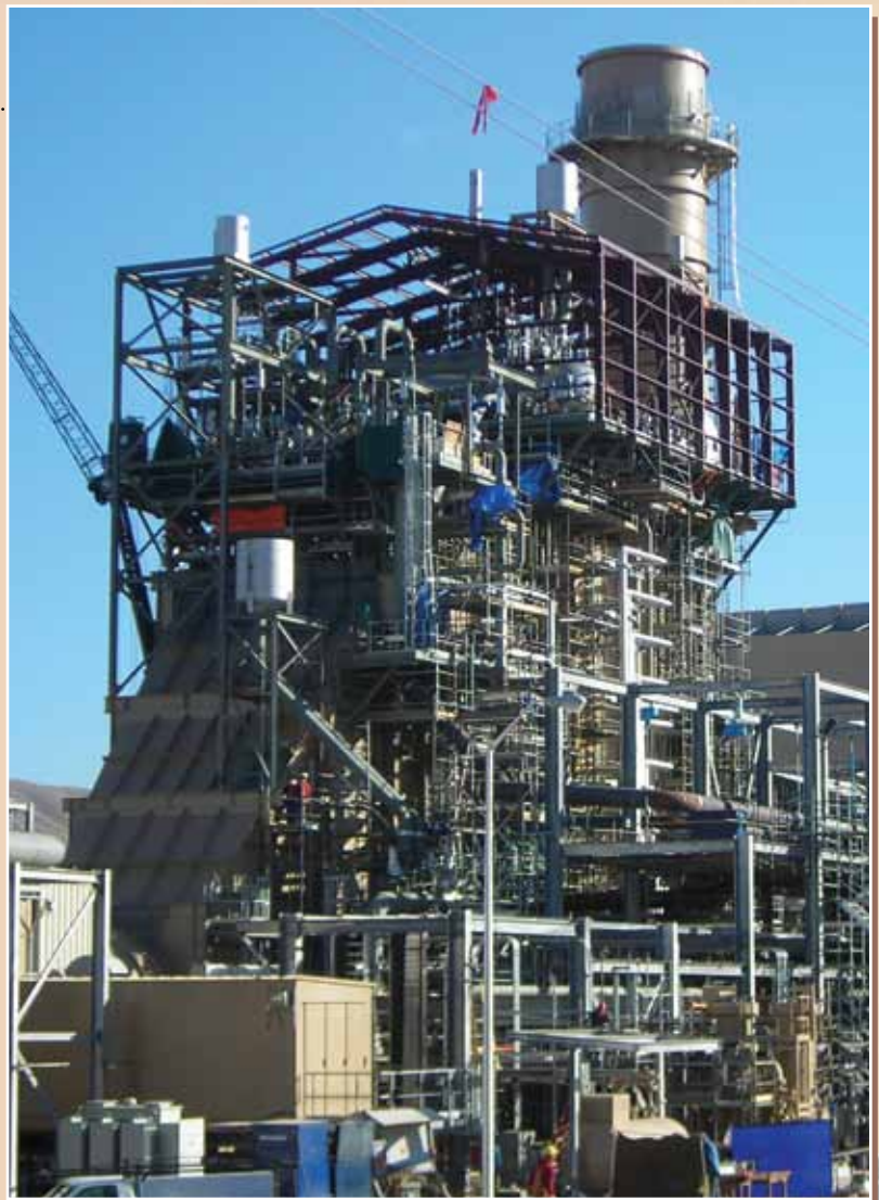
HRZG Penthouse enclosure designed, engineered and fabricated by Agate
