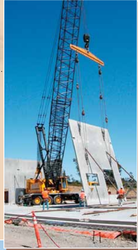
Tilt-up concrete construction provided by Agate
